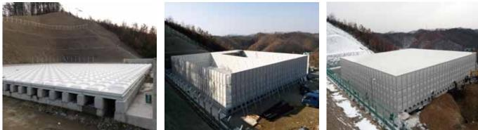
**Base Concrete** PAD & Bottom Panel assembly
